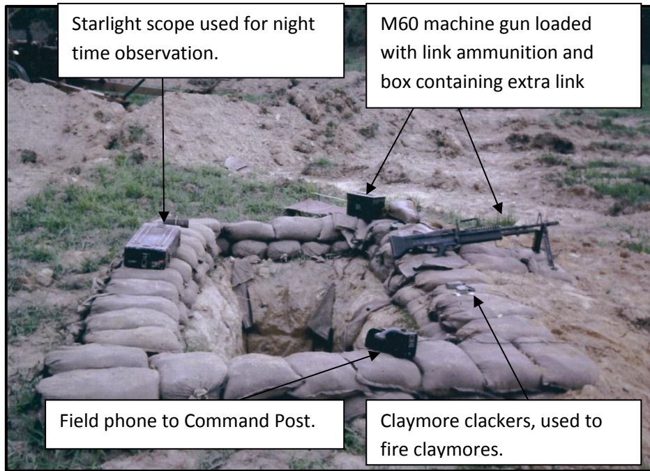
Above, M60 gun pit in the process of being completed with all the additional equipment that was required. It generally took two men to work on the gun pit along with some help from the dozer to push the dirt around. The hole was dug by hand making it pretty tough going in the beginning. Below Tomo, Cossie and Larry awaiting fire orders at unknown FSPB.
